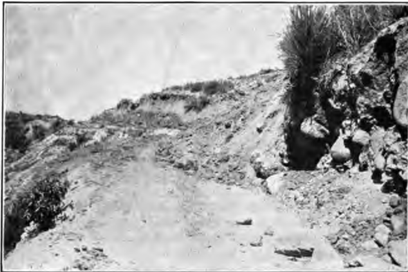
FIG. 12. THE ROAD BETWEEN HEMET AND IDYLWILD, CALIFORNIA, BLOCKED BY LANDSLIDES IN THE EARTHQUAKE OF APRIL 21, 1918 (Photograph by Homer Hamlin.)
