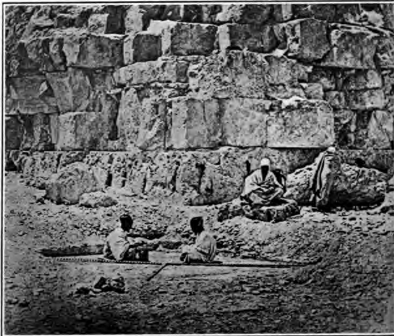
FIG. 69. RECTANGULAR SOCKET CUT IN THE NATIVE ROCK UNDERLYING THE GREAT PYRAMID. In this socket the northeast corner-stone of the building was laid; it was carried off by the Moslems.
