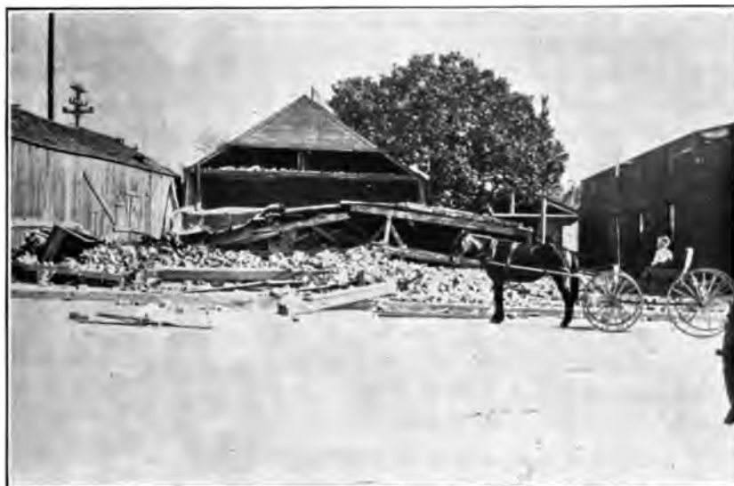
FIG. 13. BUILDINGS IN THE BUSINESS DISTRICT OF SAN JACINTO, CALIFORNIA, WRECKED IN AN EARTHQUAKE ON APRIL 21, 1918. (Photograph by Homer Hamlin.)
