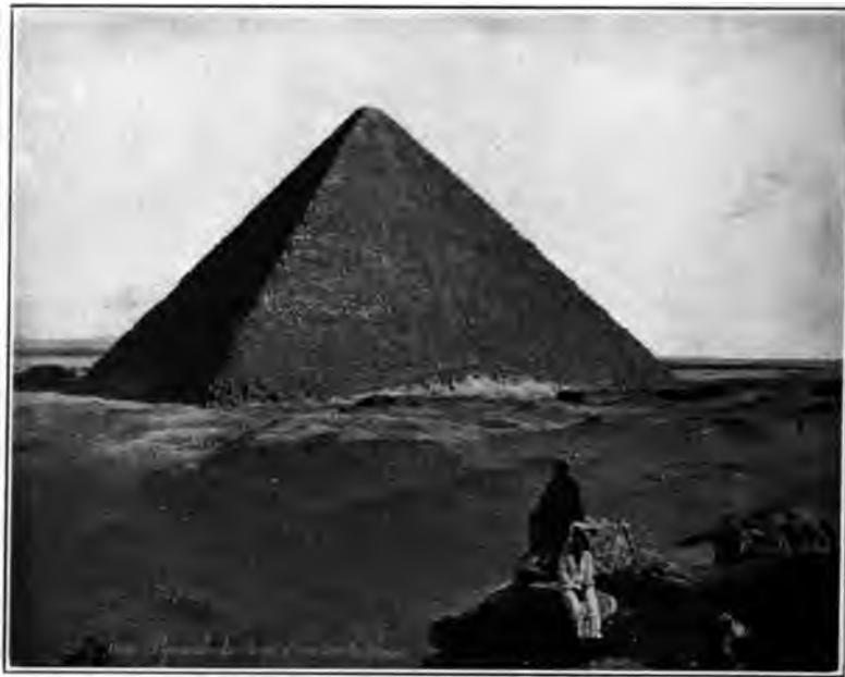
FIG. 68. THE GREAT PYRAMID OF GIZEH, THE TOMB OF THE PHARAOH KHUFU (CHEOPS), BUILT IN THE TWENTY-NINTH CENTURY B.C. It is the largest stone superstructure ever erected whether in ancient or (except recently) in modern times.
