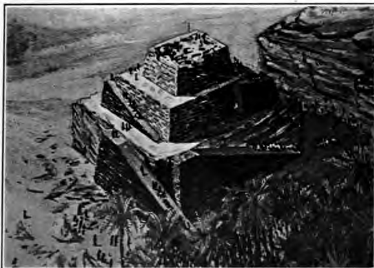
FIG. 70. UNFINISHED PYRAMID AT GIZEH, SHOWING SUN-DRIED BRICK RAMPS FOR CARRYING UP BUILDING MATERIAL. (Restored after Hoelscher.)
