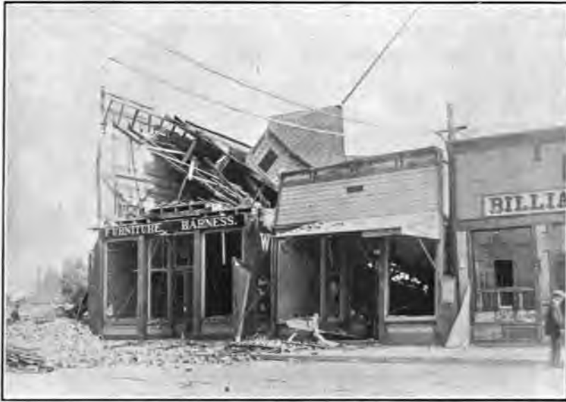
FIG. 11. A PHOTOGRAPH TAKEN IN THE BUSINESS DISTRICT OF SAN JACINTO, CALIFORNIA, FOLLOWING THE EARTHQUAKE OF APRIL 21, 1918. The center building was the telephone office. Note the difference in the damage sustained by the brick and the frame buildings here shown. (Photograph by S. D. Townley.)
