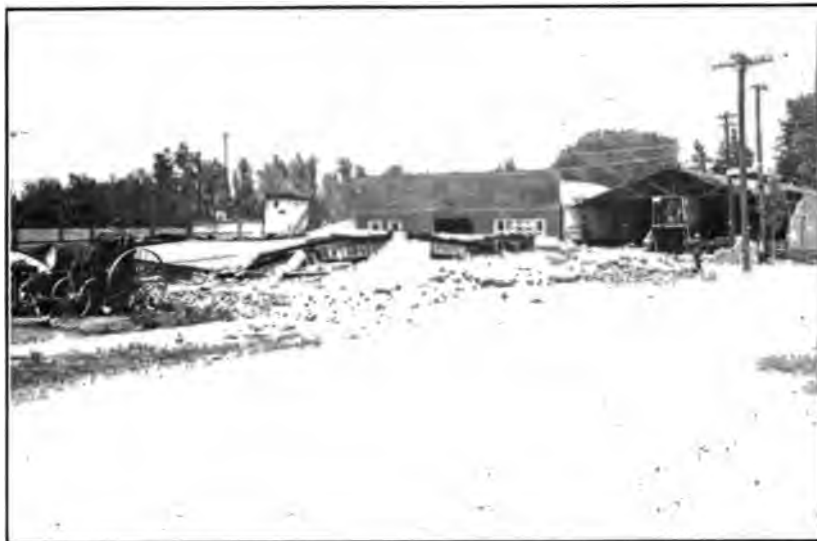
FIG. 7. BUSINESS HOUSES IN SOUTHERN CALIFORNIA LEVELLED TO THE GROUND IN A SEVERE EARTHQUAKE, WHICH CAUSED A PROPERTY LOSS ESTIMATED AT $300,000. (Photograph by Homer Hamlin.)
