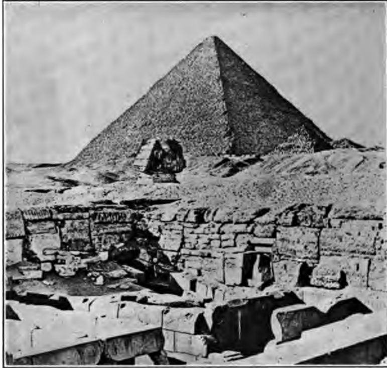
FIG. 79. INCIPIENT CLERESTORY IN THE HALL OF THE VALLEY TEMPLE OF KHAFRE AT GIZEH BUILT IN THE 29TH CENTURY B.C. The narrow light-chutes occupying the difference in level between a higher roof over the nave and a lower roof beside it are the lineal ancestors of the clerestory windows of European architecture. The oblique light which they admit is seen in Fig. 80.
