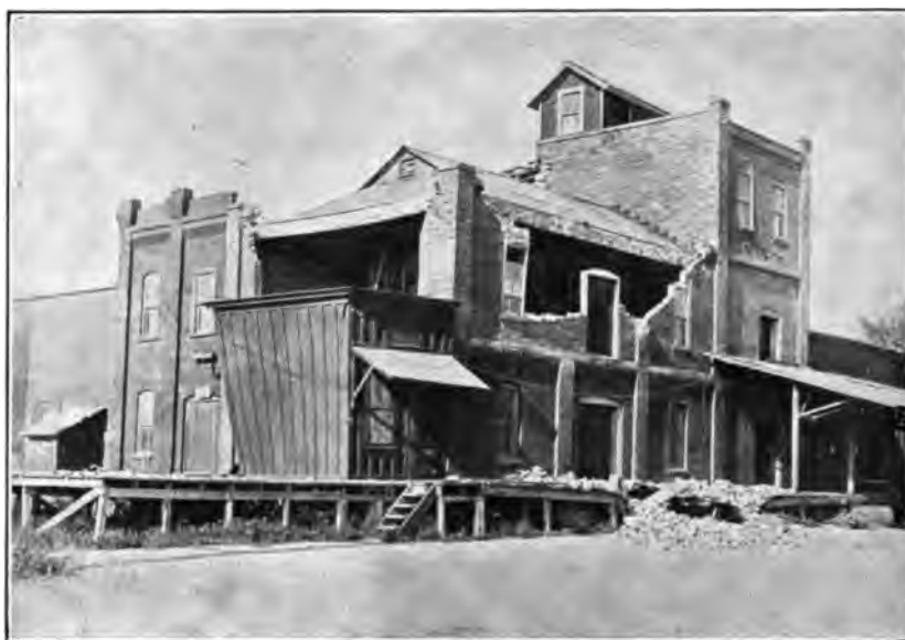
FIG. 4. A VIEW OF A FLOUR MILL AT HEMET, CALIFORNIA, SHORTLY AFTER THE EARTHQUAKE OF APRIL 21, 1918. Brick and adobe buildings can not withstand severe earthquakes, whereas reinforced concrete and steel frame buildings will stand through the strongest shocks. (Photograph by S. D. Townley.)
