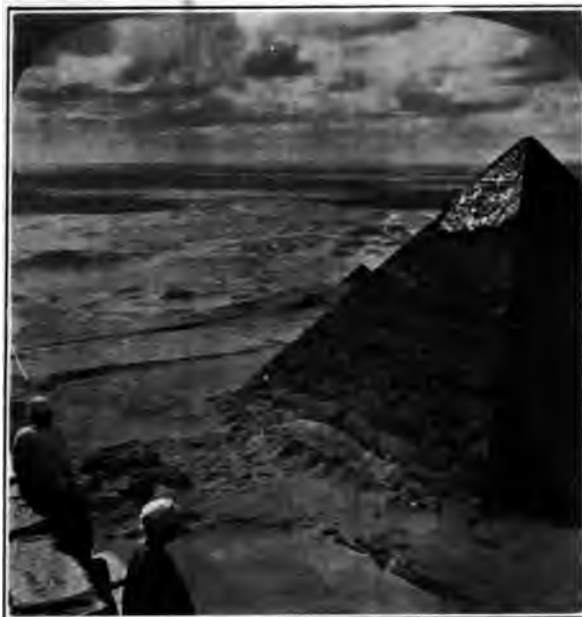
FIG. 76. SECOND PYRAMID OF GIZEH, BUILT BY KING KHAFRE IN THE 29TH CENTURY B.C. A bonnet of casing masonry is still preserved at the summit; below on the left we discern the ruins of the pyramid-temple described in the text and shown in Fig. 79. (By Underwood & Underwood, Copyright.)
