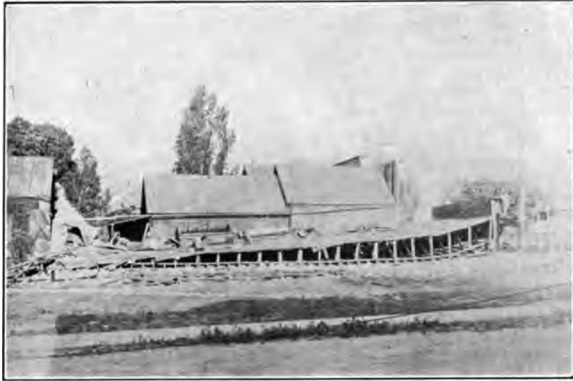
FIG. 15. A BUILDING ON MAIN STREET, SAN JACINTO, CALIFORNIA, WRECKED IN AN EARTHQUAKE ON APRIL 21, 1918. (Photograph by Homer Hamlin.)
