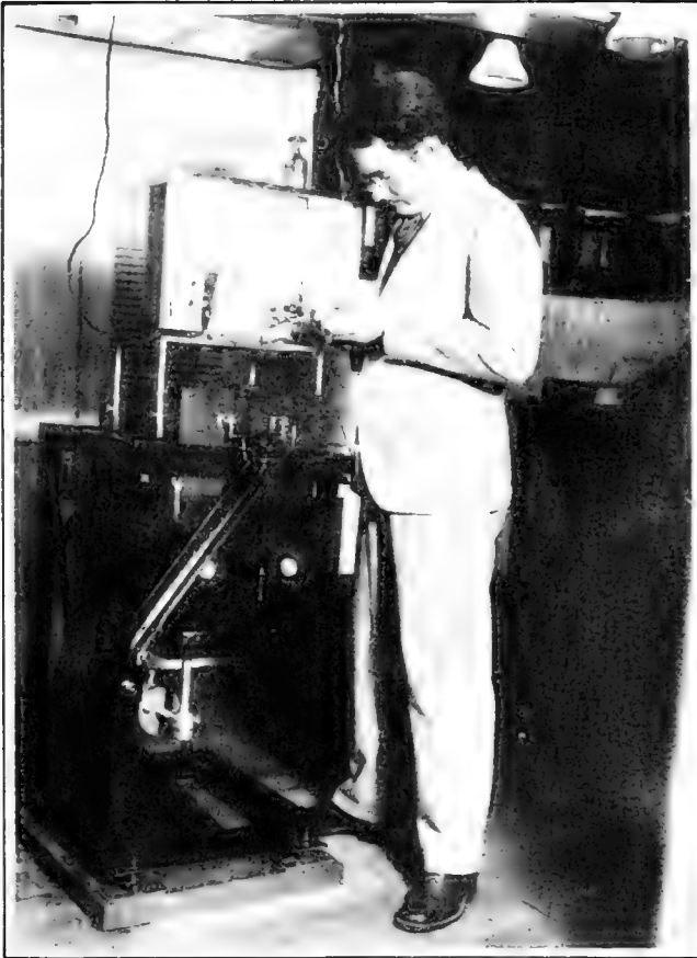
Fig. 1. Vening-Meinesz gravity instrument installed in the main cabin of the Carnegie
