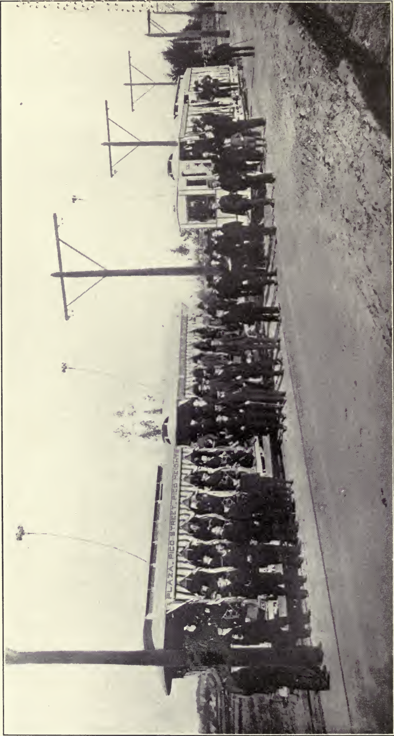
Fig. 1. The first electric locomotive built in the United States is here shown drawing two trailers, also the first over-head wire system for trolley cars which was constructed in Los Angeles, California, in 1886.
