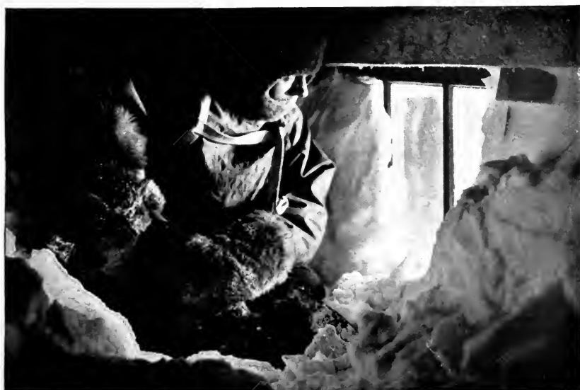
CLEARING DRIFT FROM WINDOW OF HUT AT CAPE ADARE
