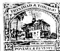
Town Hall, San Fernando A9
