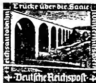
Bridge over the Saale, Saxony SP82
