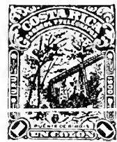
Birris Bridge A36
