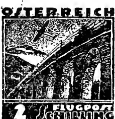
Airplane over R. R. Viaduct at Karnten AP16
