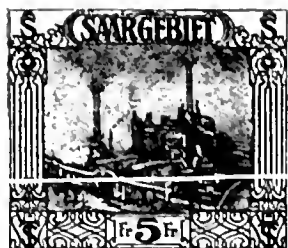
Blast Furnaces at Dillingen A29
