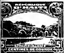
Aqueduct at Prince A53
