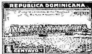
Trujillo Bridge A41
