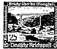
Bridge over the Mangfall SP84
