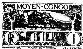
Viaduct at Mindouli A4
