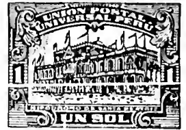
Grandstand at Santa Beatriz Race Track A43
