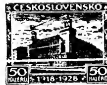
Telephone Exchange at Praha A21
