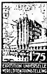
Belgian Building A79
