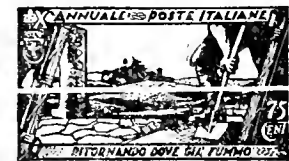
Excavating Ruins A155
