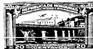
Mayol Bridge AP7
