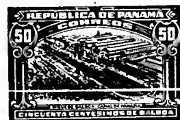
Dry Dock at Balboa A38
