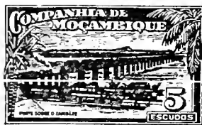
Zambezi Railroad Bridge A52
