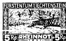
R. R. Bridge Demolished by Flood SP3
