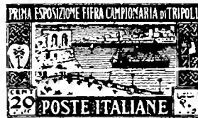
View of Port Tripoli SP11
