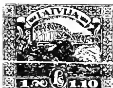
Riga Bridge and Trenches SP13
