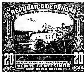
Madden Dam, Panama Canal A73
