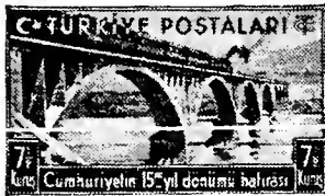
Railway Bridge A99
