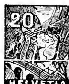
Saint Gotthard Railroad A50
