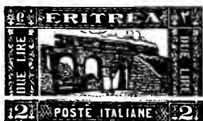
Railroad Viaduct A37
