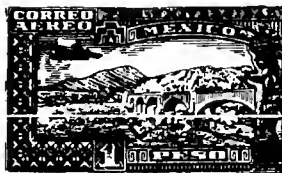
Bridge over Tepecayo AP11
