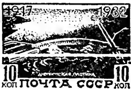
Dnieper Hydroelectric Power Station A136
