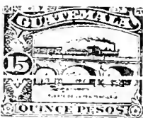
"Penitenciaria" Bridge A64
