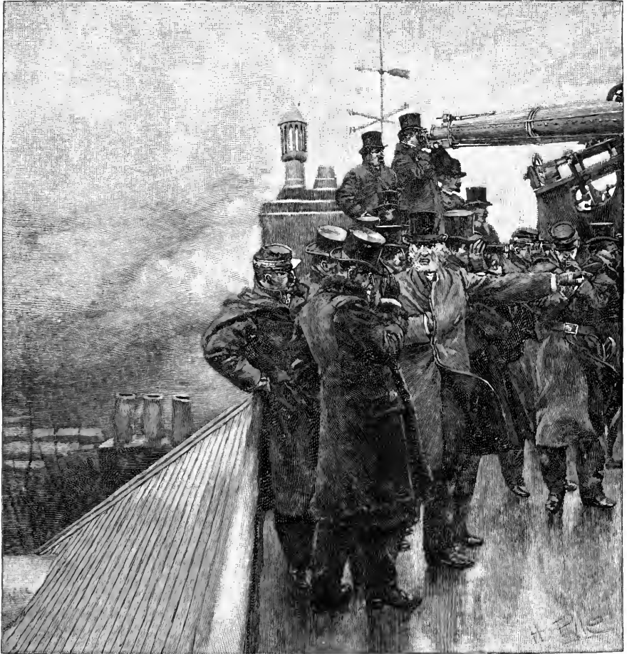
Looking into the Prussian Lines from the Château de la Muette.
