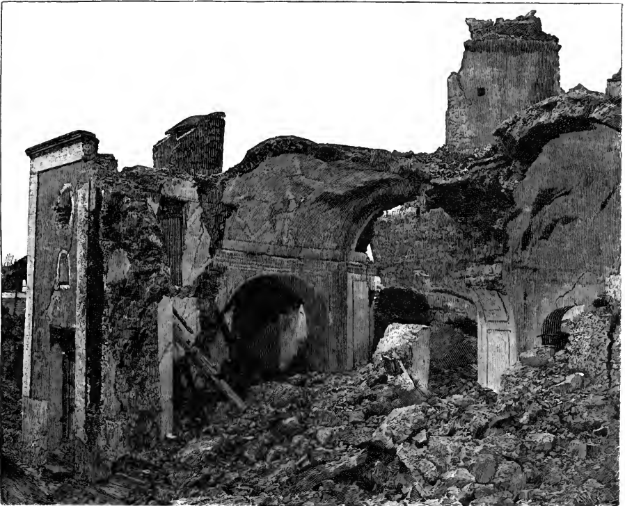
Effect of a Powerful Earthquake on Massive Masonry, Italy.
