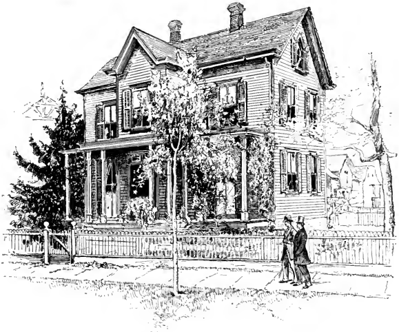
House of a Western Union Telegraph Superintendent at Mount Vernon, N. Y., cost $2,200, exclusive of ground.
