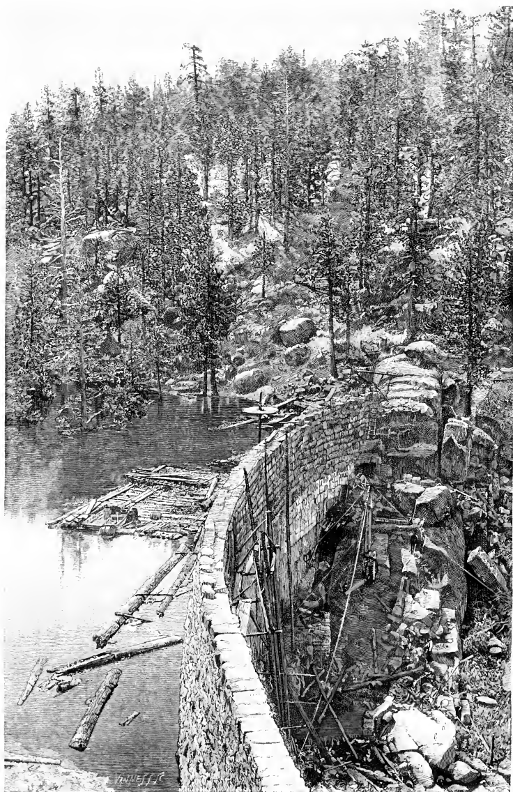
DAM ACROSS THE BEAR VALLEY, SAN BERNARDINO COUNTY, CAL.
