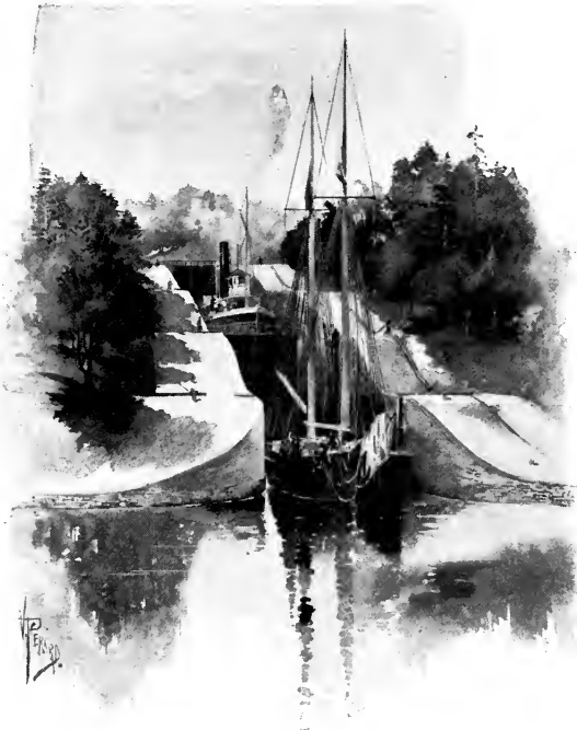
Lock on Götha Canal, Trollhattan Falls.
