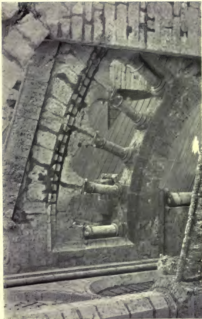
39. Flying buttresses of the Nave.
