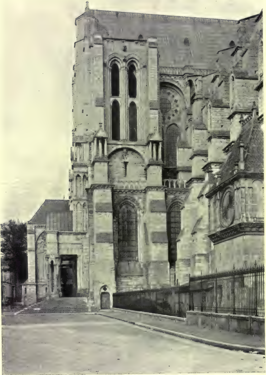
38. North Transept. Transept nord.
