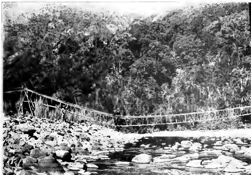
Fig. 2. Rattan bridge built by Mangyans, near Sablayan.
