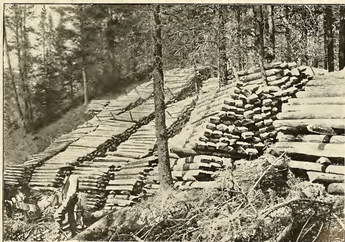
FIG. 2.—TIE PILES AT THE FLUME.
