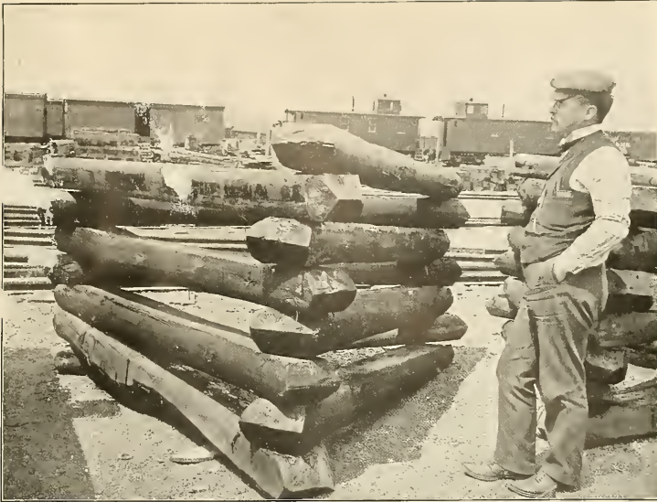
FIG. 1.—TRIANGULAR TIE PILES.
