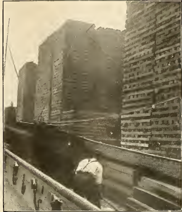
FIG. 2.—PILING BALTIC PINE ON THE GREAT WESTERN RAILWAY, ENGLAND.
