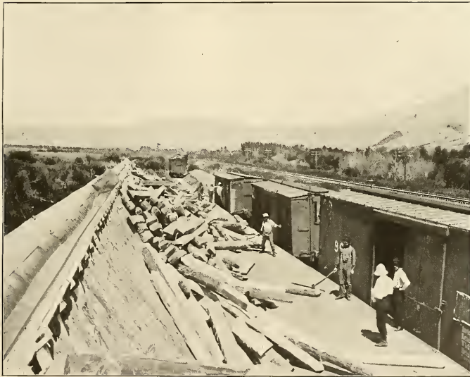
FIG. 2.—ANOTHER VIEW OF LANDING PLATFORM.
