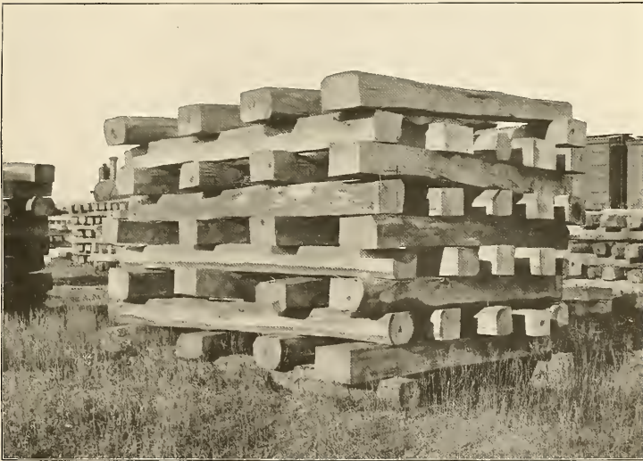
FIG. 2.—ANOTHER OPEN-CRIB PILE.
