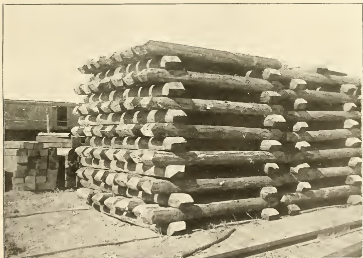
FIG. 2.—AFTER TREATMENT. LOGGEPOLK PINE, OPEN-CRIB PILE.
