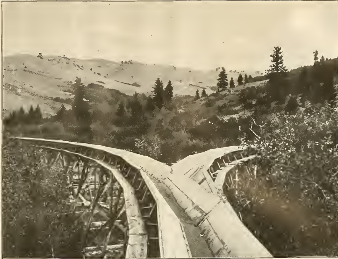
FIG. 1.—END OF FLUME AT RAILROAD TRACK.
