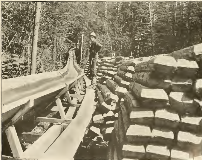
FIG. 2.—TIES READY FOR THE FLUME.
