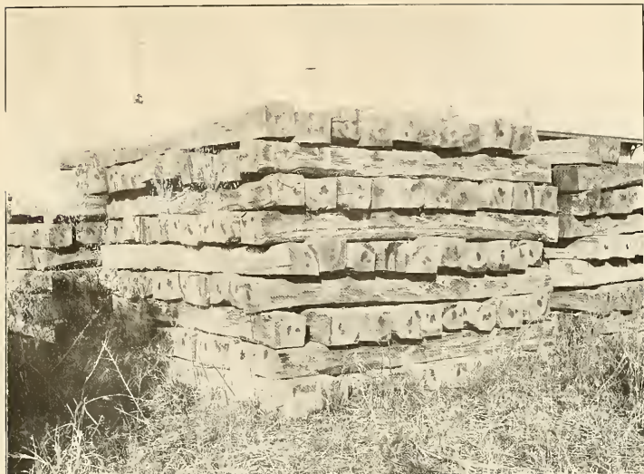
FIG. 1.—OAK PILES, SHOWING LOWEST TIER ON THE GROUND—A POOR METHOD.
