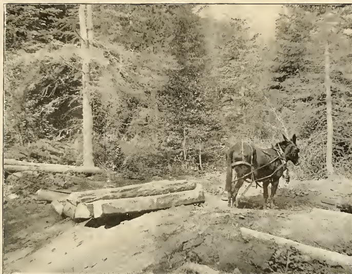
FIG. 1.—DRAGGING TIES TO THE FLUME.
