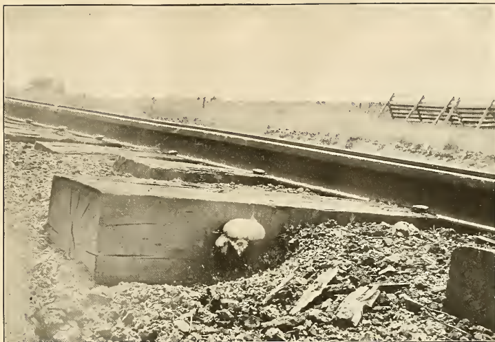
FIG. 1.—FRUITING BODY OF FUNGUS ON TIE IN POSITION.
