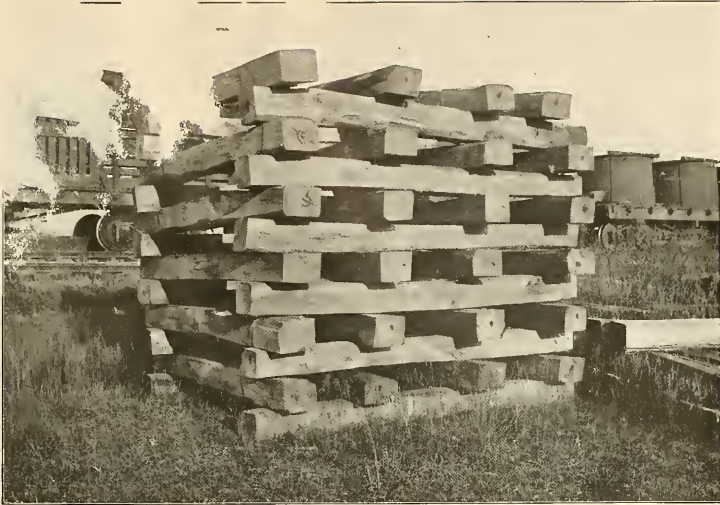
FIG. 1.—OPEN-CRIB OAK PILE, SOUTHERN ILLINOIS.
