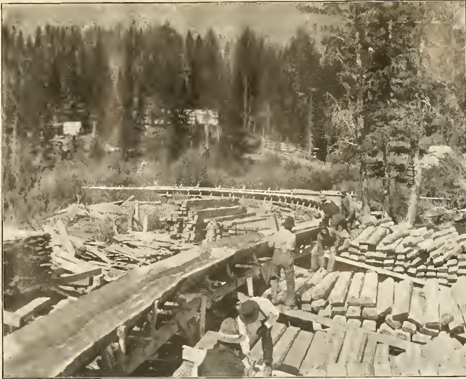
FIG. 1.—THROWING TIES INTO THE FLUME.
