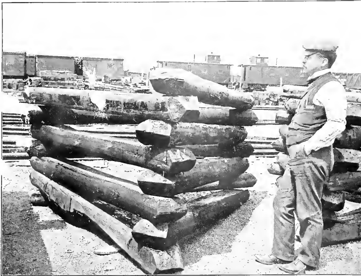
FIG. 1.—TRIANGULAR TIE PILES.
