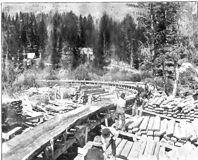
FIG. 1.—THROWING TIES INTO THE FLUME.
