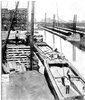
FIG. 3.—TIES ARRIVING IN CANAL BOATS, GREAT WESTERN RAILWAY, ENGLAND.
