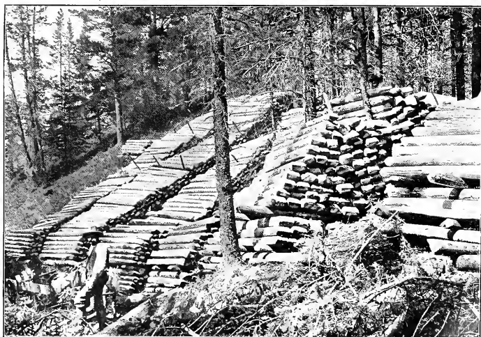
FIG. 2.—TIE PILES AT THE FLUME.
