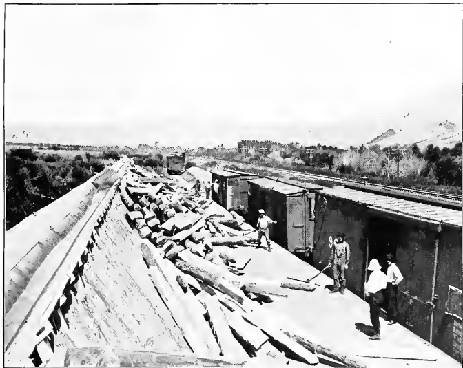
FIG. 2.—ANOTHER VIEW OF LANDING PLATFORM.
