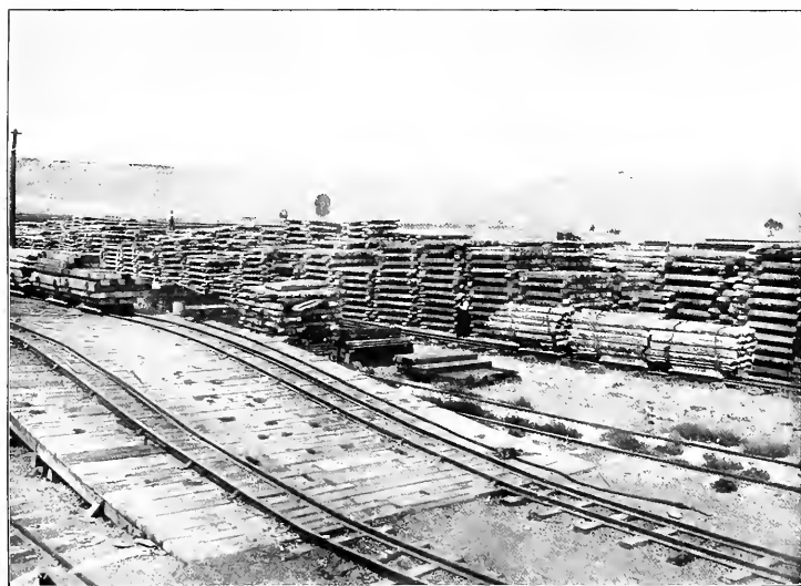
FIG. 2.—TIE YARD, SHERIDAN, WYO., SEPTEMBER, 1902—OPEN PILES.
