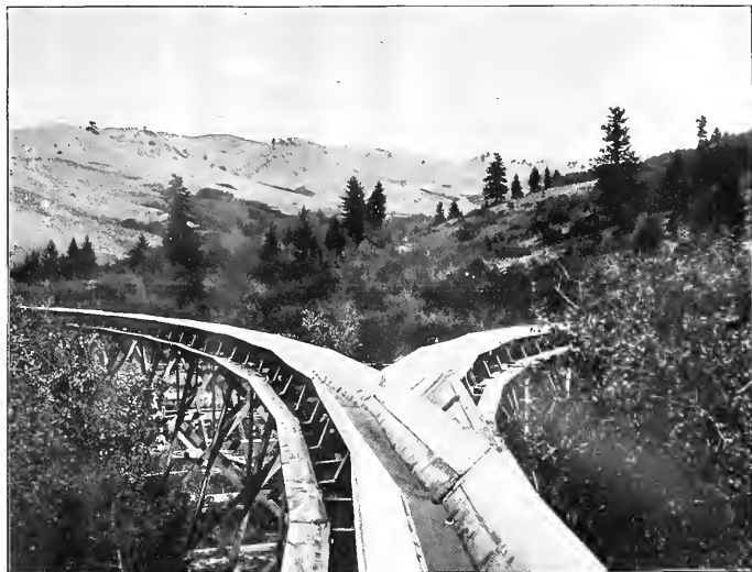
FIG. 1.—END OF FLUME AT RAILROAD TRACK.
