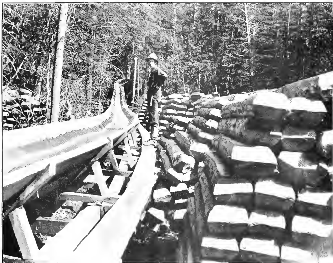
FIG. 2.—TIES READY FOR THE FLUME.
