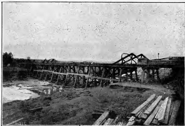
TEMPORARY BRIDGE AT FRERE.— Engineering.
