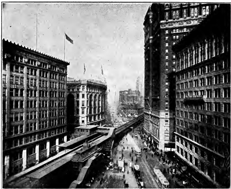
THE TRAIN THAT TRAVELS OVERHEAD
