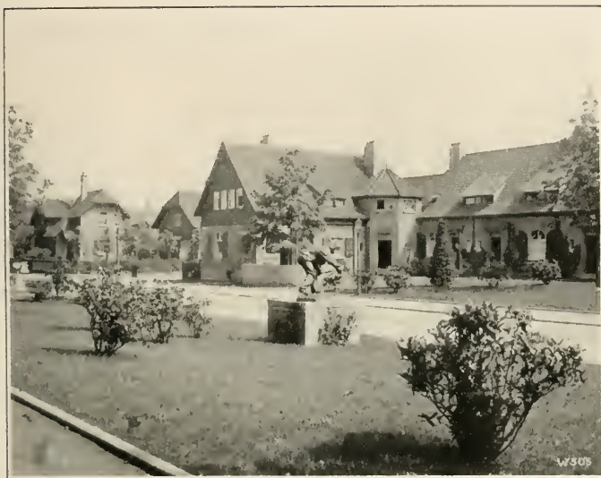
Street in Workingmen's Colony, Altenhof.
