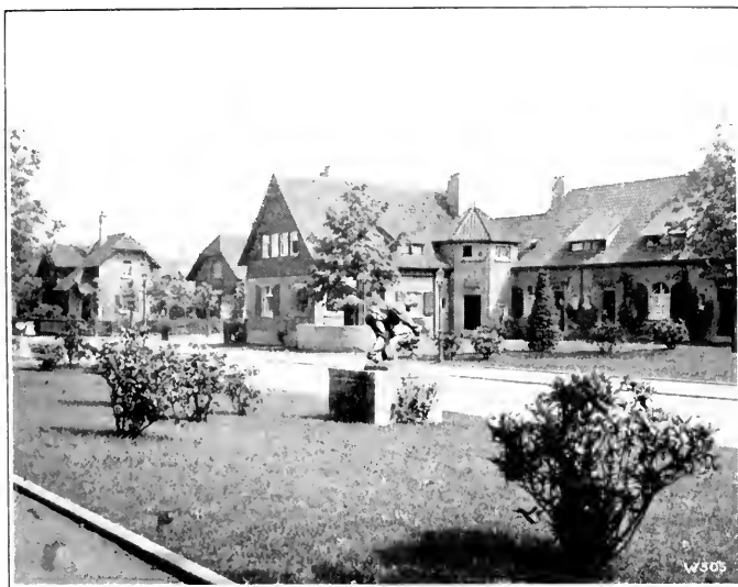
Street in Workingmen's Colony, Altenhof.
