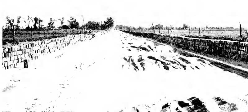
ROAD FROM WICHITA TO WACO, CONCRETE WITH BRICK PAVING (In Construction)
