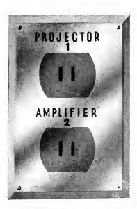
Outlet C above. One side of this 110 volt A.C. outlet connected to control panel (D) in front of the room
