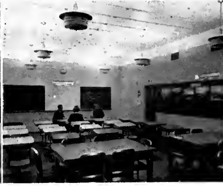
Plate 2. Classroom demonstration in second phase, using indirect fixtures.
