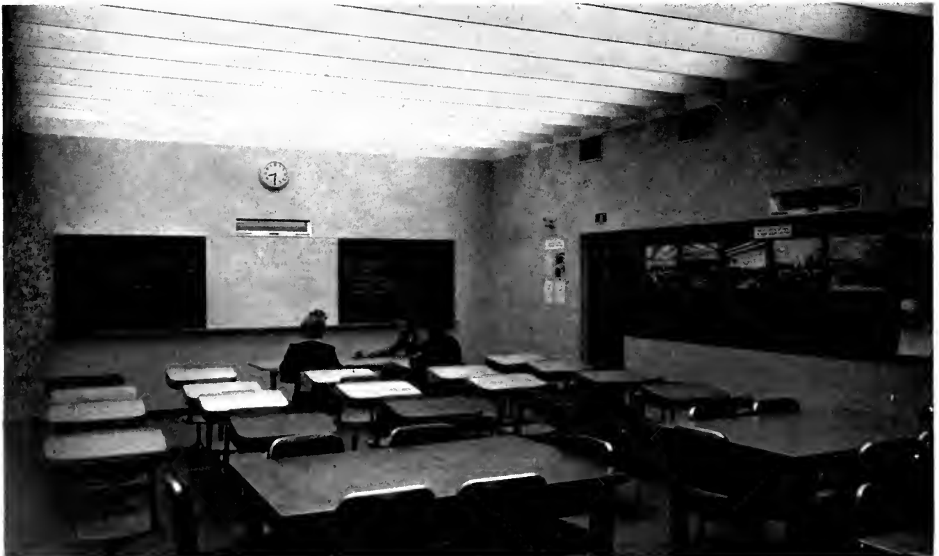
Plate 4. Fourth phase of model classroom lighting demonstration showing use of vertical shields between lamps.
