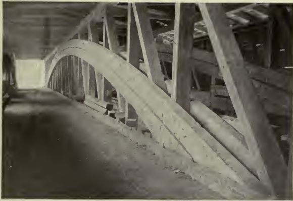
COVERED BRIDGE OVER KISKIMINETAS, NEAR SALTSBURG, PENNSYLVANIA
