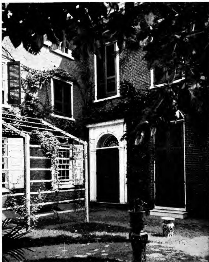
READ HOUSE, NEW CASTLE, DELAWARE From the Garden
