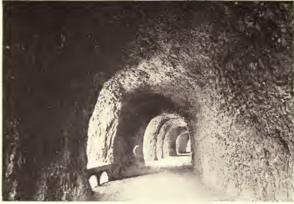
INTERIOR OF MITCHELL'S POINT TUNNELS, COLUMBIA RIVER HIGHWAY, SHOWING "THE FIVE WINDOWS"
