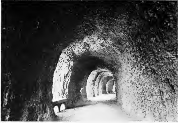
INTERIOR OF MITCHELL'S POINT TUNNELS, COLUMBIA RIVER HIGHWAY, SHOWING "THE FIVE WINDOWS"
