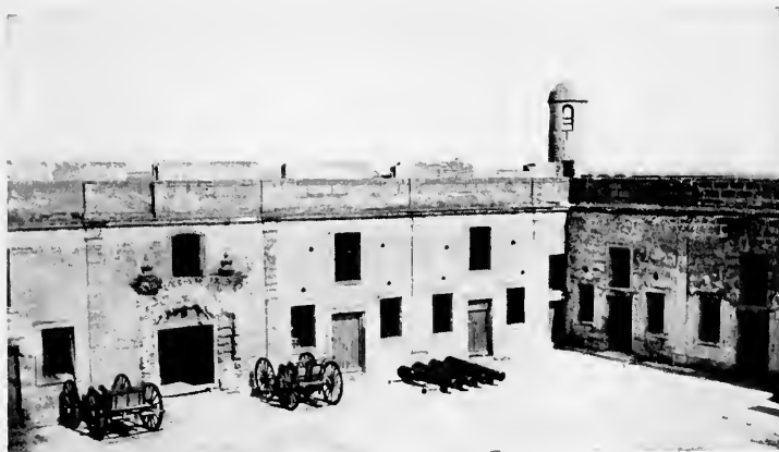
WITHIN THE WALLS OF FORT MARION, ST. AUGUSTINE, FLORIDA
