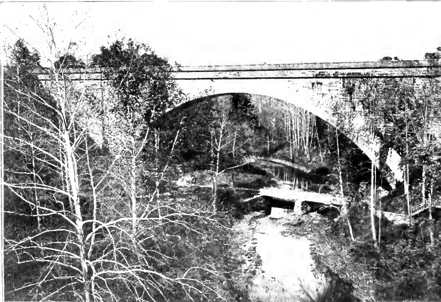
CABIN JOHN BRIDGE. ONE OF THE LARGEST SINGLE SPANS OF MASONRY IN THE WORLD. OVER CABIN-JOHN RUN.
