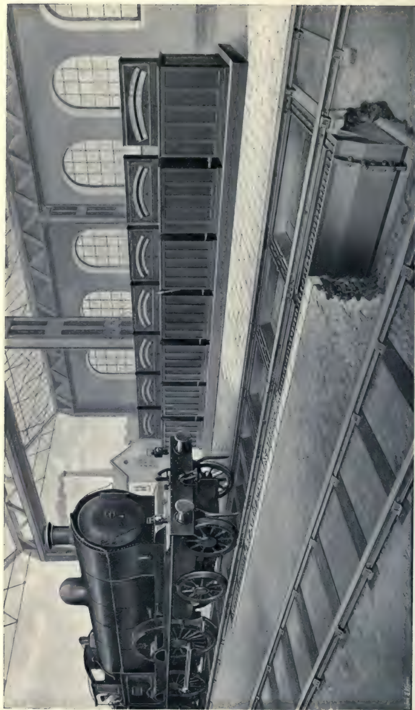
Locomotive Engine Weighing Tables with Avery's "Aerostat" Indicating Quadrants.
