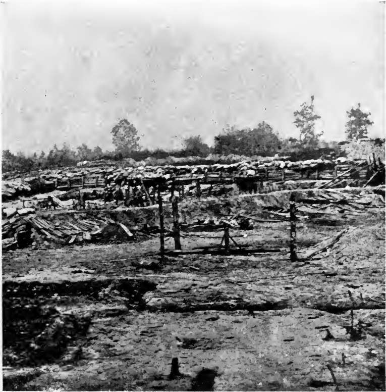
WORKS AT PRIEST CAP, PORT HUDSON
