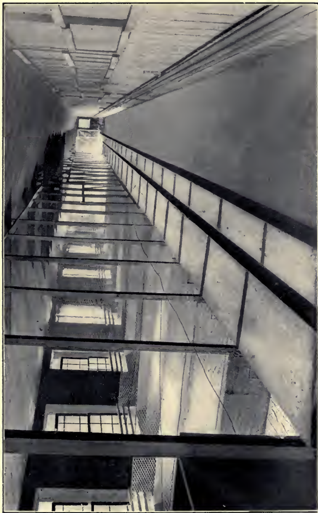
INTERIOR OF SECTIONAL BROODER HOUSE ONE HUNDRED FEET LONG, HEATED BY HOT WATER, USED ON LARGE BROILER PLANTS
