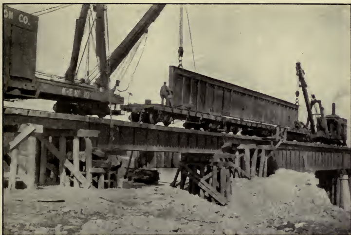
Students of engineering help build bridges
