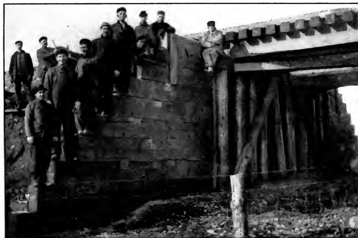
Future engineers work on section gangs
