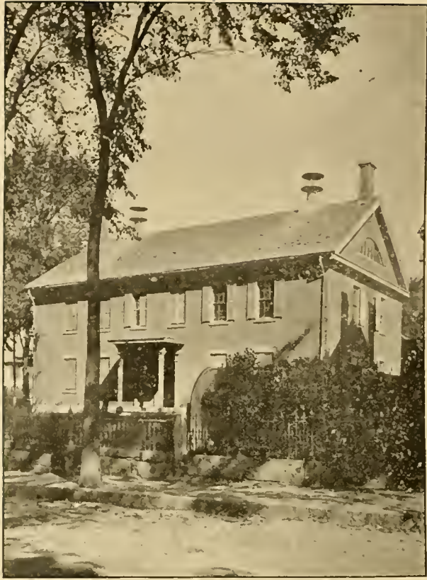
FIRST BRICK SCHOOLHOUSE. ERECTED 1841.
