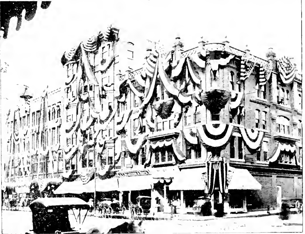
W. RESTON, HILL & FITZ AND GILLEY BUILDINGS.
