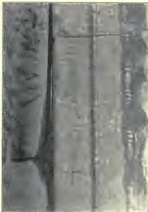
Jamb in East Church at Ksēdjbeh.
