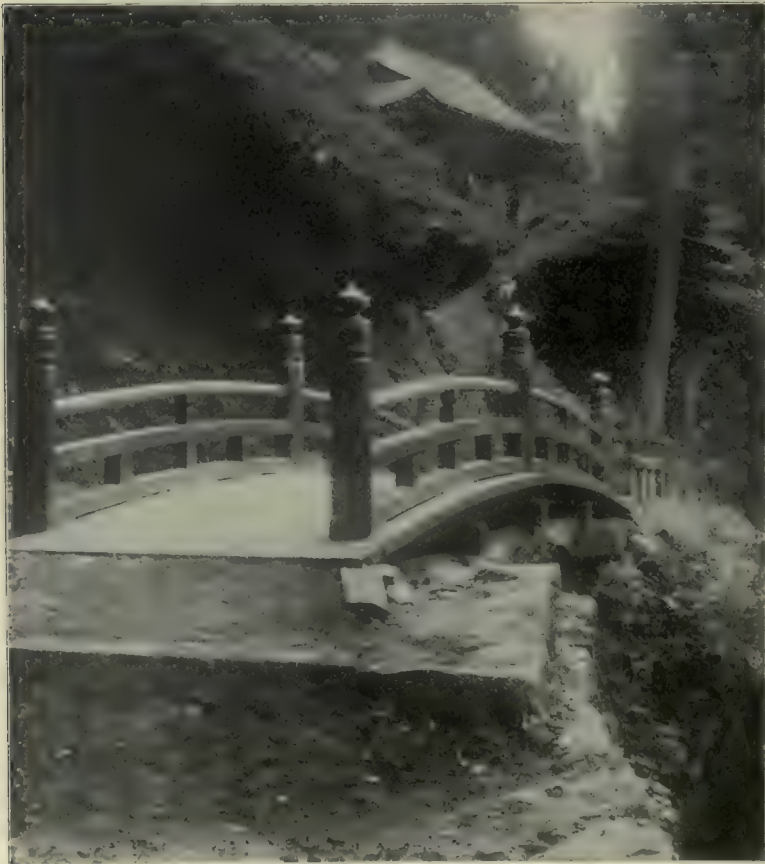
A BRIDGE AT HARUNA
