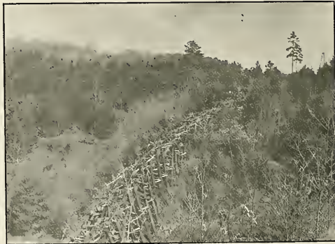
A Wrecked Trestle Near Clarion
