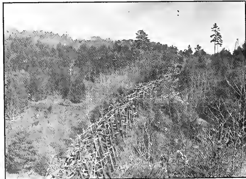
A Wrecked Trestle Near Clarion
