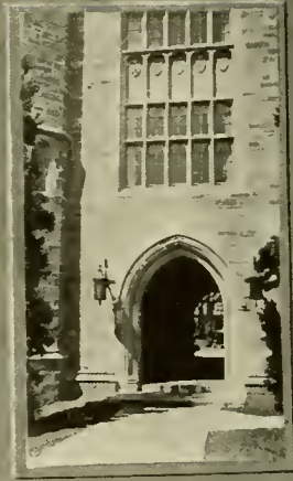
Philips Memorial Building
