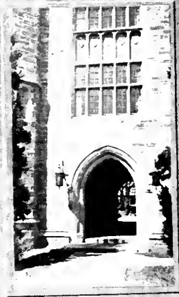
Philips Memorial Building
