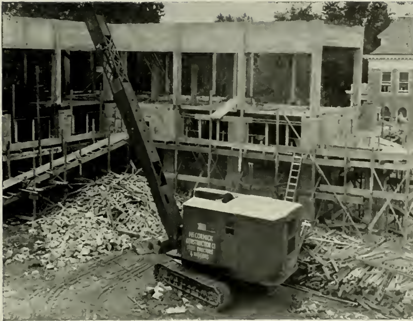
While the girders were being put in place, construction was delayed by a general strike. This picture was taken sometime after operations were resumed.
