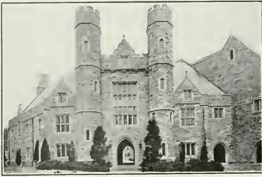
Philips Memorial Building
