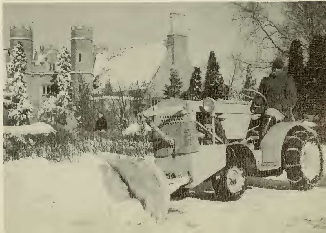
A cold job for this member of the Maintenance Department!
