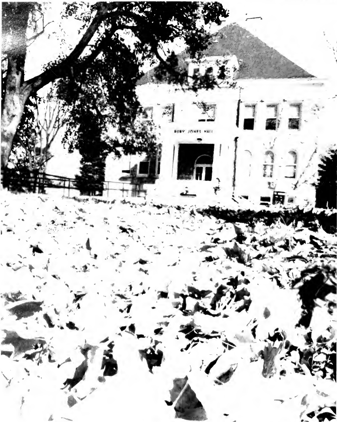
Ruby Jones Hall, built in 1899, adds beauty and history to the WCU campus.
