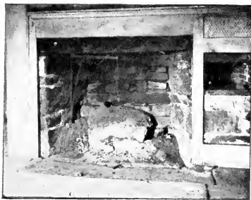
FIRE-PLACE IN HOUSE OF ALEXANDER JOHNSON.
