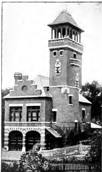
THE ENGINE HOUSE.
