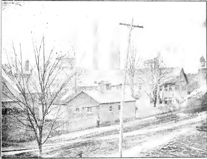
THE FOWLER NAIL CO'S WORKS.
