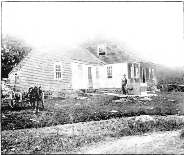
THE WEST END OF THE GUNN-NETTLETON-SCRANTON HOUSE
