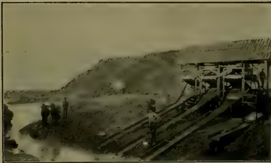
Watsonville plant of Pacific Coast Chemical Gold Mining Co., Watsonville, Cal., U. S. A.
