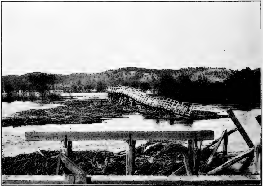
Broken Bridge at Eagle Point above Dubuque.
