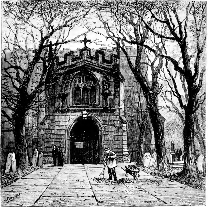
PORCH, STRATFORD CHURCH
