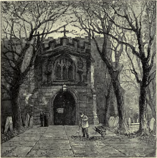
PORCH, STRATFORD CHURCH
