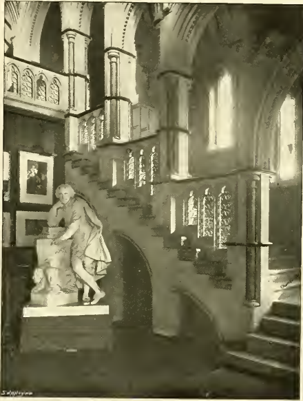
STAIRWAY, MEMORIAL LIBRARY.
