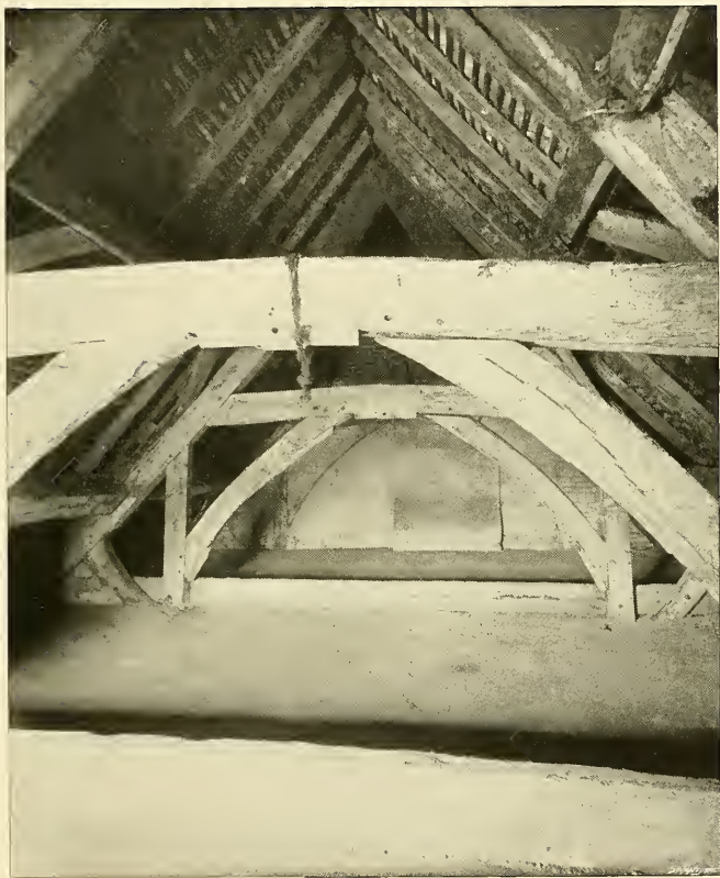
THE ROOF ROOM, SHOTTERY MANOR.
