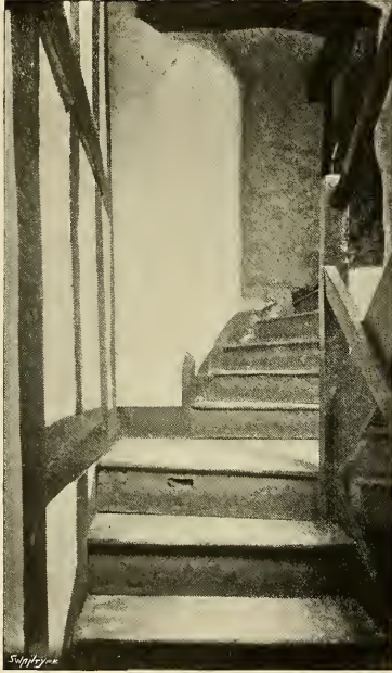
STAIRS TO THE MUNIMENT ROOM, GUILD HALL.
