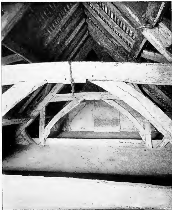
THE ROOF ROOM, SHOTTERY MANOR.
