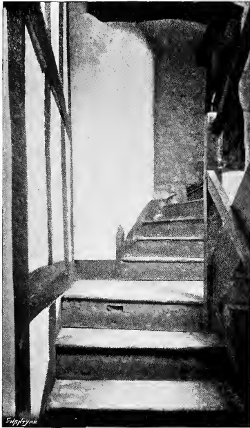
STAIRS TO THE MUNIMENT ROOM, GUILD HALL.
