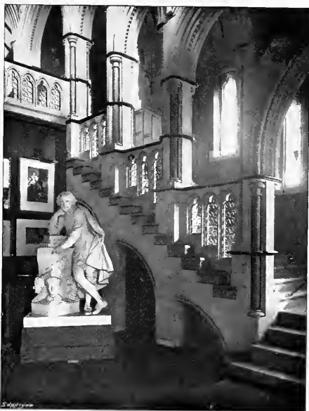
STAIRWAY, MEMORIAL LIBRARY.
