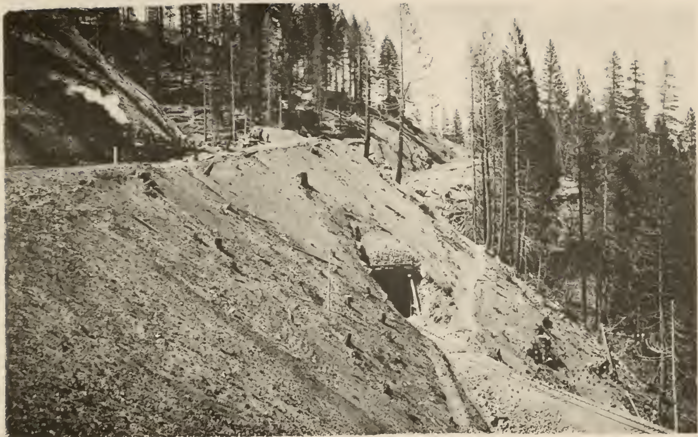
LOOP AND TUNNEL 16, SISKIYOU MOUNTAINS.
