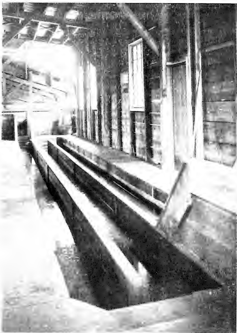
Mammoth Sheep-Dipping Vat at the New York Central Stock Yards, Buffalo, N. Y. Length of Swim in the clear 136 feet. Capacity 100 Sheep at a time. Heated by steam and with all the latest improvements, making it by far the largest and best appointed Dipping Plant in the United States.
